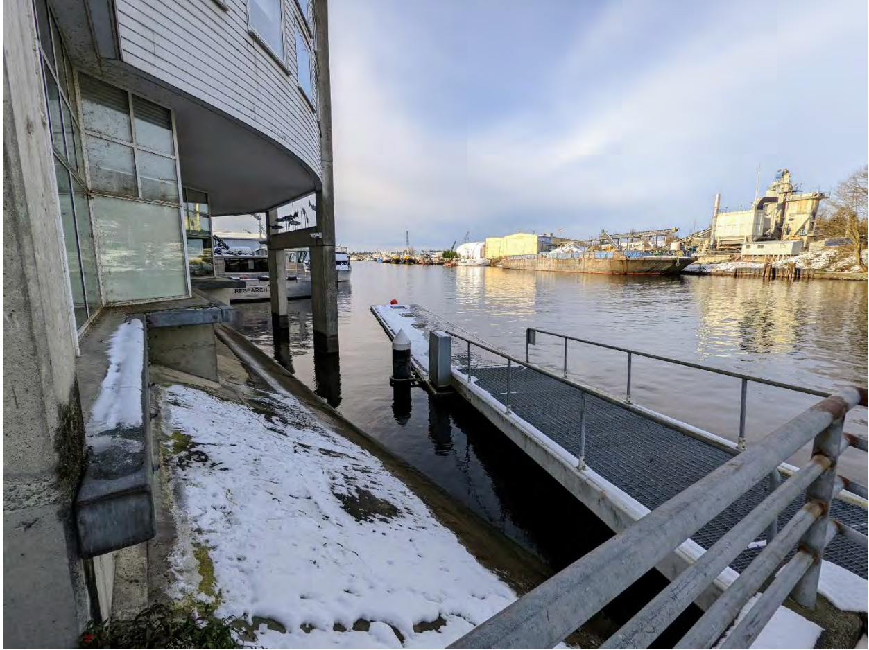
Figure 4 – King County bulkhead lease area (looking N – taken 29-DEC-2021)
