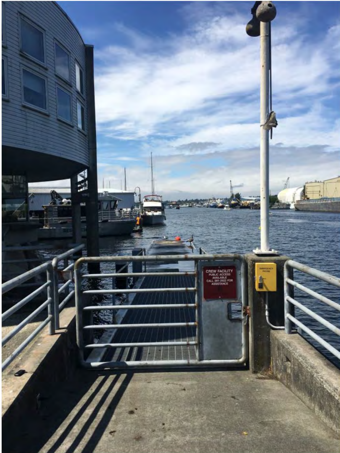
Figure 1 – King County bulkhead lease area (looking NW – taken 6-AUG-2021).
